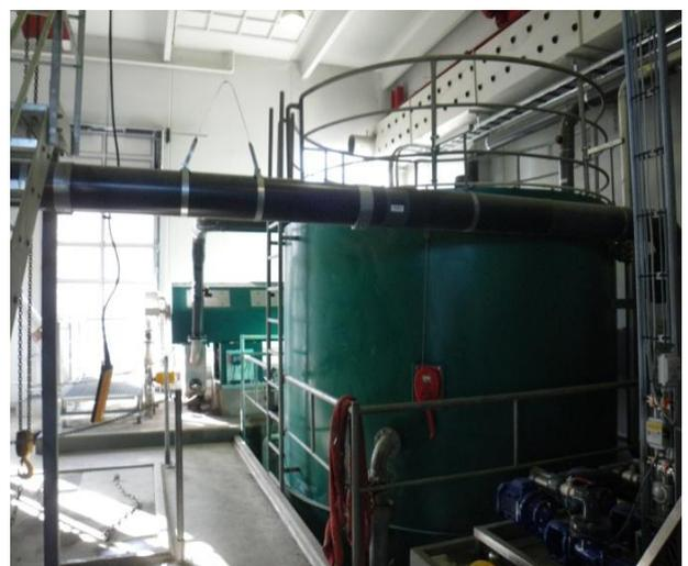
**The Installation:** municipal waste water producing 2000 to 4000 m<sup>3</sup> of treated water per hour. The treated water was discharged to the sea and bacteria count should be the same as bathing water requirements, less than 1000 CFU/100ml for *E. Coli* and less than 10000 CFU/100ml of total *Coli*.
